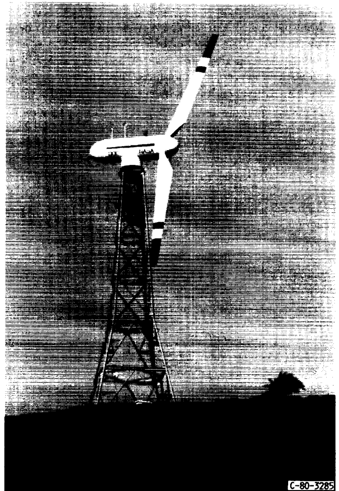
Figure 8.—DOE/NASA 200-kW Mod-0A experimental wind turbine near Kahuku Village, Oahu, Hawaii. Laminated Douglas fir/epoxy blades form the 125-ft-diameter rotor.
