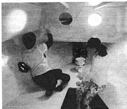
Madison and Sean Nolan putting latex house paint on the cabin. $10 a gallon. Works great over cured epoxy.
