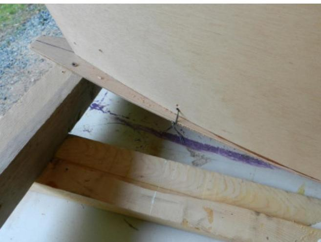
The forward bottom panel section is made overwide so you can screw it to the "spreader bar" as shown' thus stabilising and fixing the bottom point
