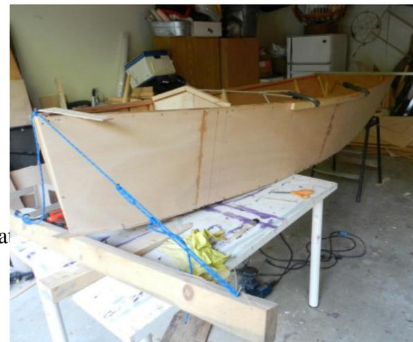
Screw a temporary spacer just aft of the stem to hold the panels together while fitting the stem (you may need help)
