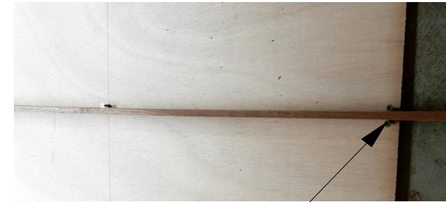
twin screws to hold batten
