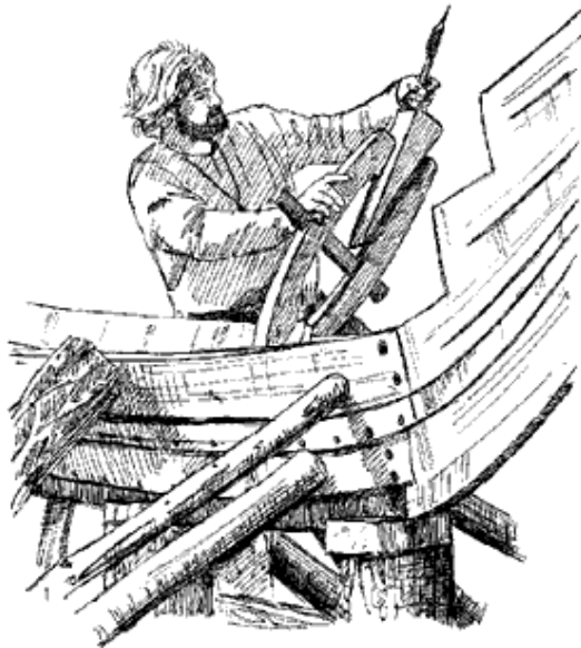
Another strake is wedged in place ready to be permanently roved onto the emerging ship.
