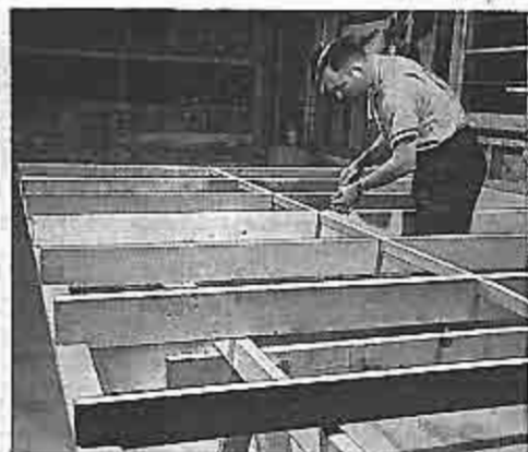
BUILDING FORM is actually just two 2 x 4 set-up rails on which the basic framing pieces are mounted
