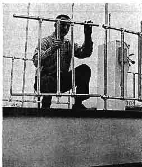
ON THE PROTOTYPE, the rails and top bows were made from aluminum assembled with NuRail fittings
