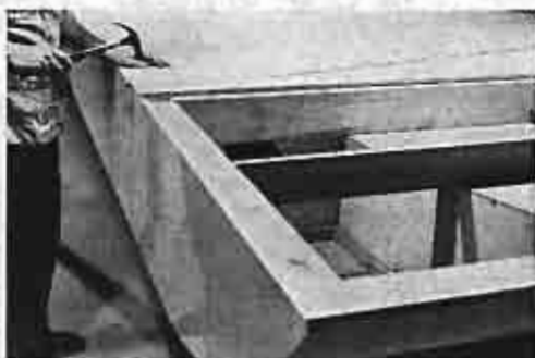
FIBERGLASS HULL before turning it over (Dynel was used here), then flip the hull and apply the decking
